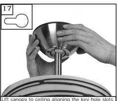
Lift canopy to ceiling aligning the key hole slots with the screws on the bottom of the mounting bracket. Rotate the canopy counter clockwise to lock in place. Tighten the screws to secure the canopy. See inset for keyhole shape
